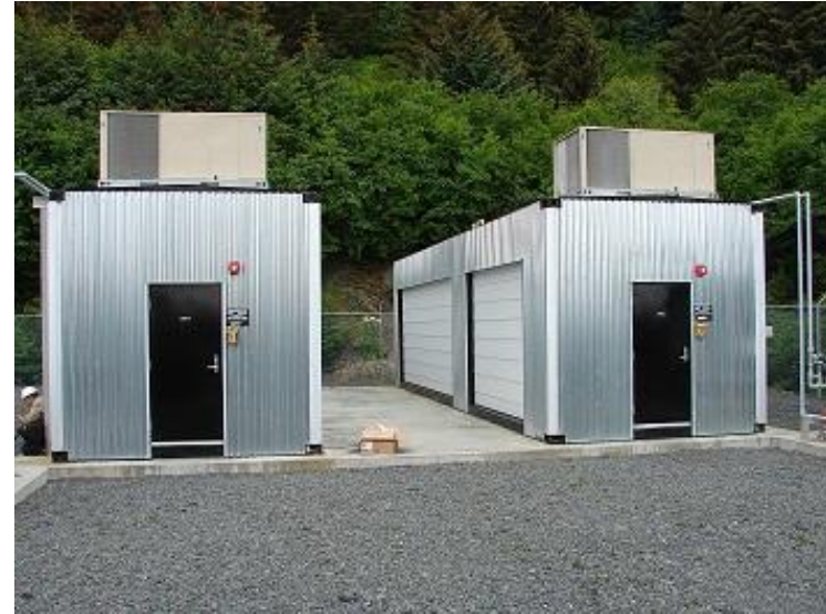
3MW site (indoor Inverters)
