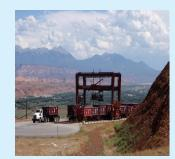
IN 2009 DOE began relocating tailings to the Crescent Junction disposal cell. Tailings are excavated and conditioned in drying beds on top of the pile to reach optimal moisture content for disposal. The tailings are then placed in steel containers with locking lids for transport. A gantry crane is used to transfer containers to and from the train at Moab.
