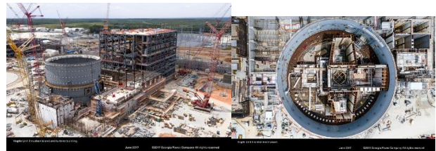
Vogtle Unit 3 Nuclear Island and Turbine Building; Vogtle Unit 4 Containment Vessel (Courtesy of Georgia Power/Southern Company; June 2017)
