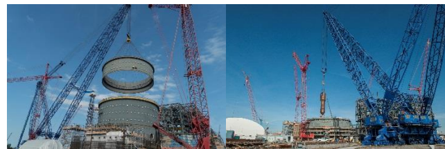
SCE&G Places Final Unit 2 Containment Vessel Ring; The First U.S. AP1000 Steam Generator is placed in Unit 2 (Courtesy of SCE&G)
