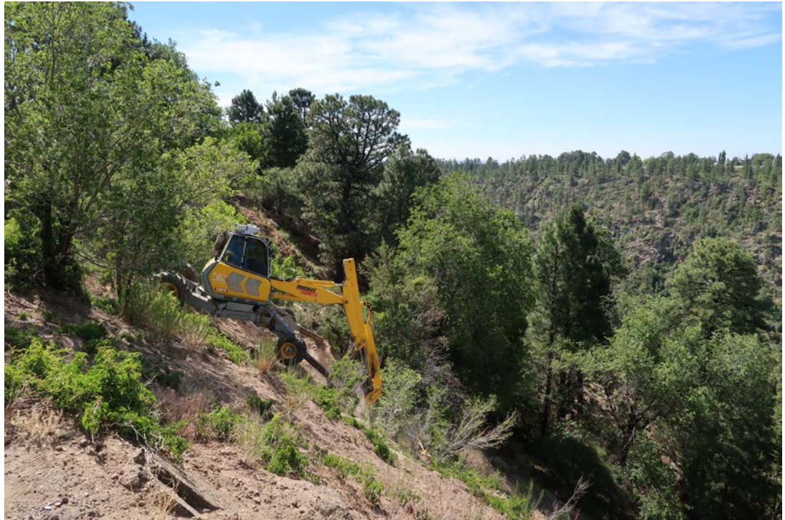
A spider excavator crawled from the canyon rim to the side of the canyon, where the second of two cleanups was completed.
