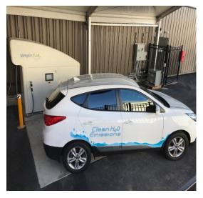
The eye-catching, seven-foot long SimpleFuel<sup>™</sup> enclosure houses all the equipment necessary to convert water into hydrogen fuel. It can be used in a variety of settings: homes, municipalities, or small businesses, and is gaining widespread industry attention. Modular fueling projects like this are integral to the deployment of hydrogen infrastructure across the country, supporting more transportation options for American consumers.
