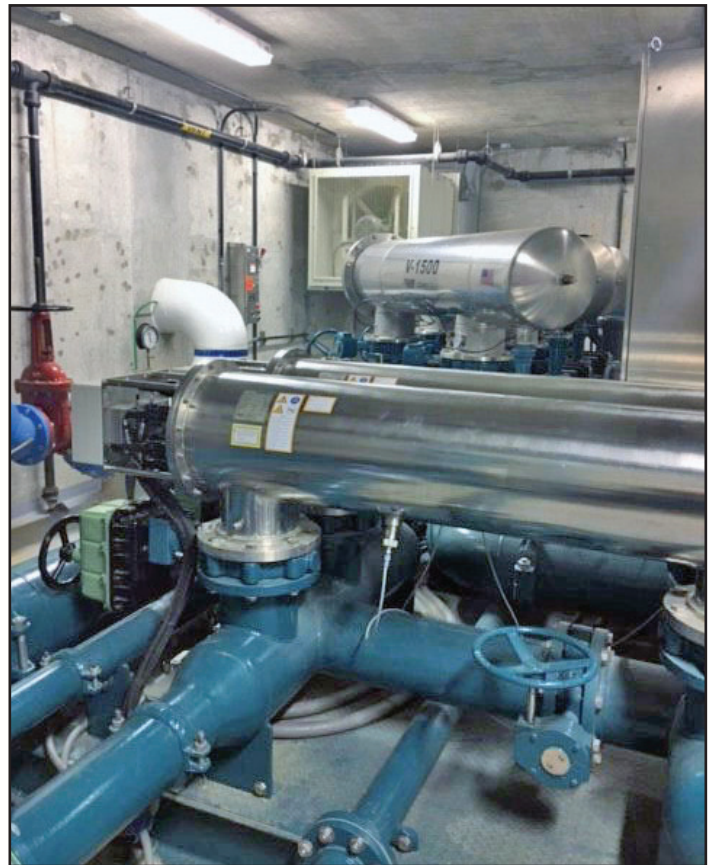
A water pump system that sits underneath the National Mall.
