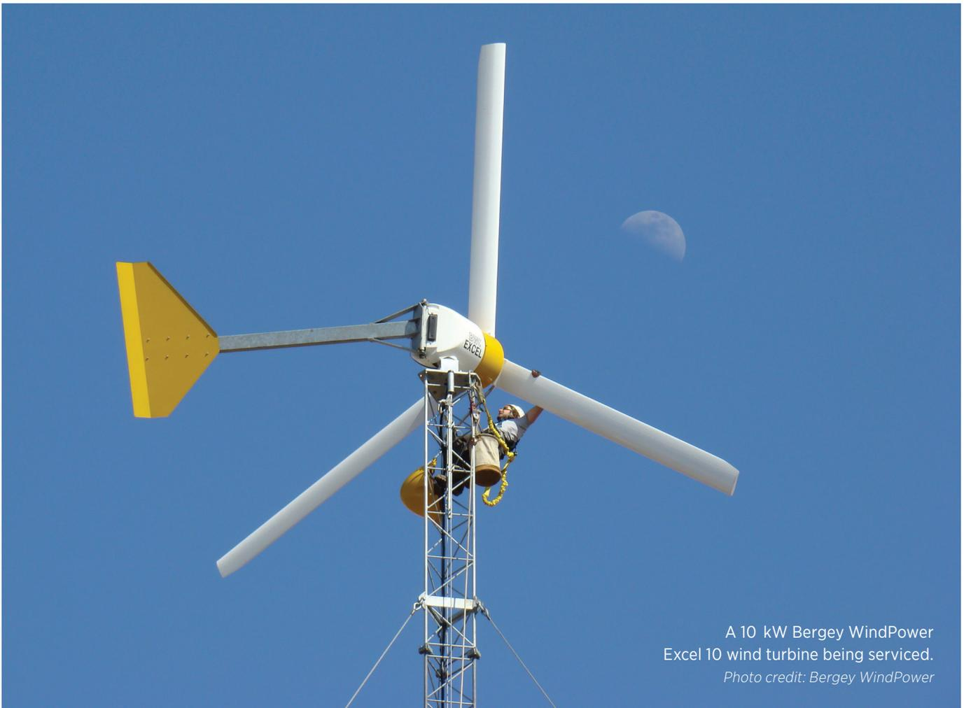
A 10 kW Bergey WindPower Excel 10 wind turbine being serviced.
