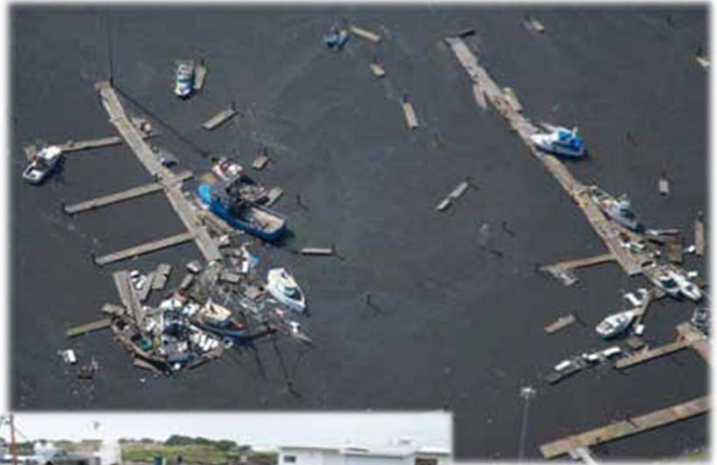
2011 Fukushima tsunami at Crescent City, CA
