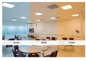
The heart of the NICLS technology is an LED module consisting of separate assemblies of warm-white and cool-white LEDs. Together with sensors and a controller, the NICLS fixtures form a made-in-USA system operated from a user interface that's either mounted in the front of a classroom or accessed
