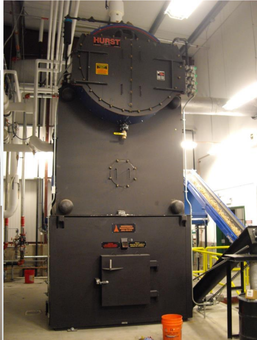
Tok School Wood-Fired Boiler
