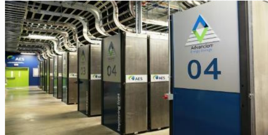
80KW ADVANCION NODE: Impact on a 40MW resource
