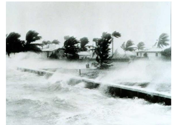
Wind-driven waves and storm surge threaten to inundate homes in Miami, Florida - 1945
