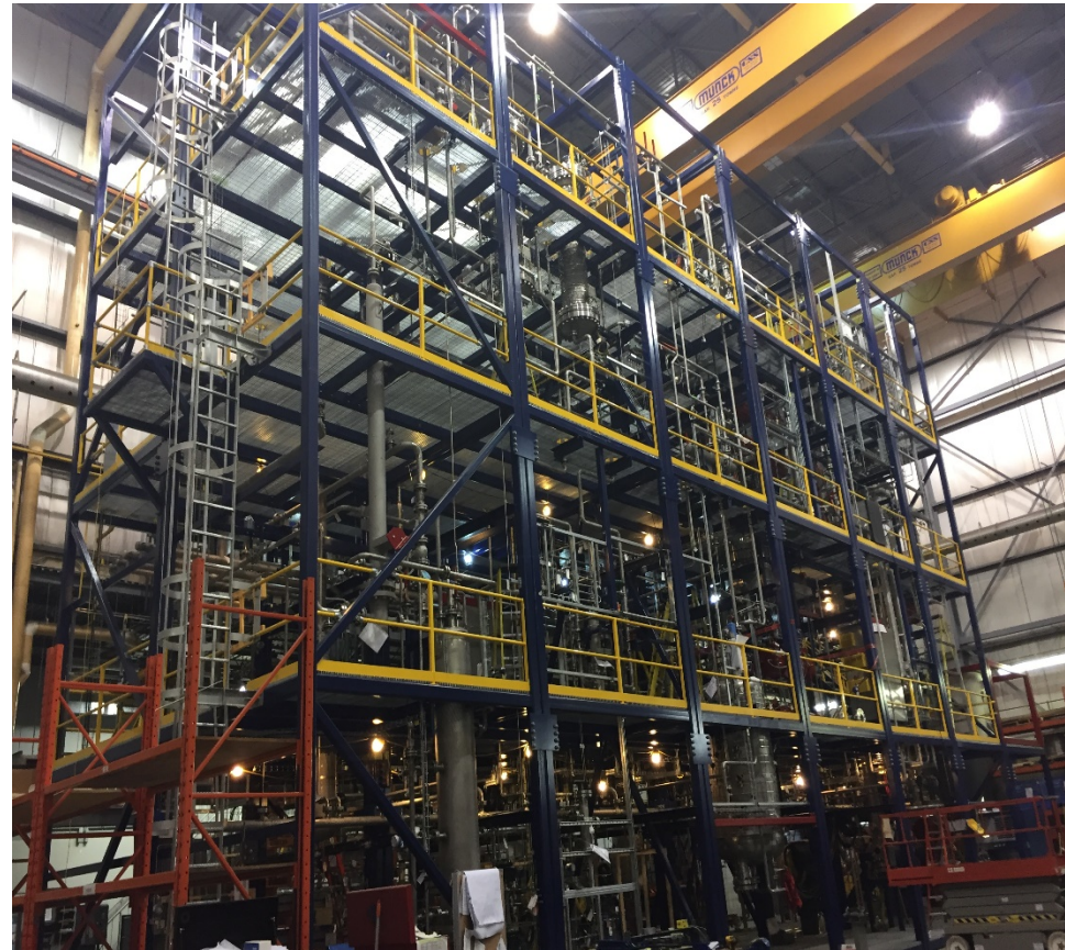
IH 2 ® 5t/day Demonstration Plant
