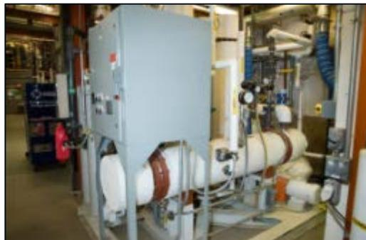
Existing atmospheric pressure evaporator is being converted to vacuum operation to reduce sugar degradation losses.
