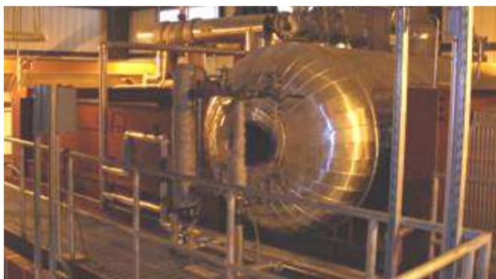
The 60,000 lb/hr stoker-fired biomass boiler serves the process and building steam demand at Frito-Lay’s Topeka, Kansas, food processing facility. *Photo courtesy of Frito-Lay, Inc.*
