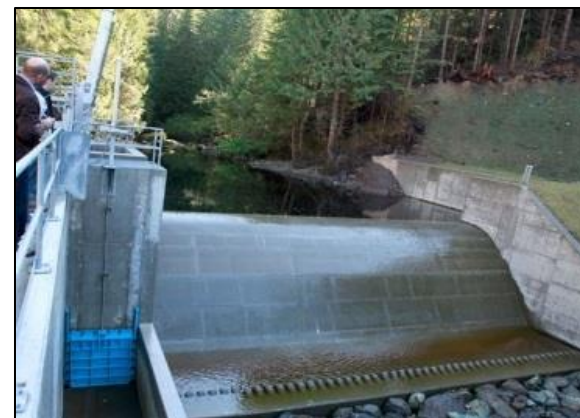
Young's Creek Hydro Project in Washington State, 2011 (7.5MW)
