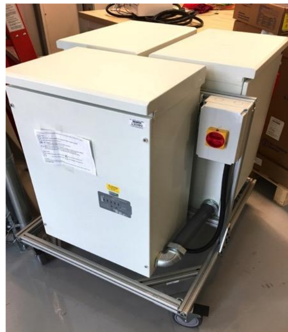
12 kWh Battery pack w/ 5-kW inverter
