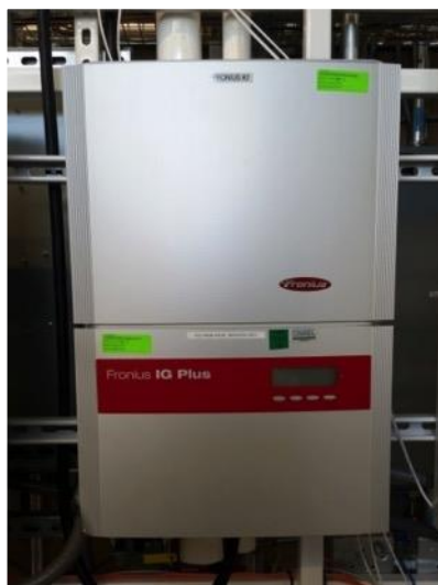
3-kW PV inverter
