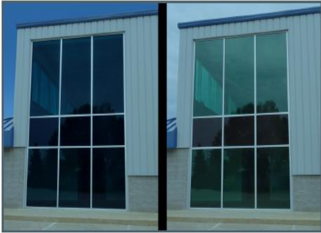
Pleotint's Suntuitive Thermochromic Interlayer Combined with PPG's Azuria Tinted Glass in the Dark and Light States
