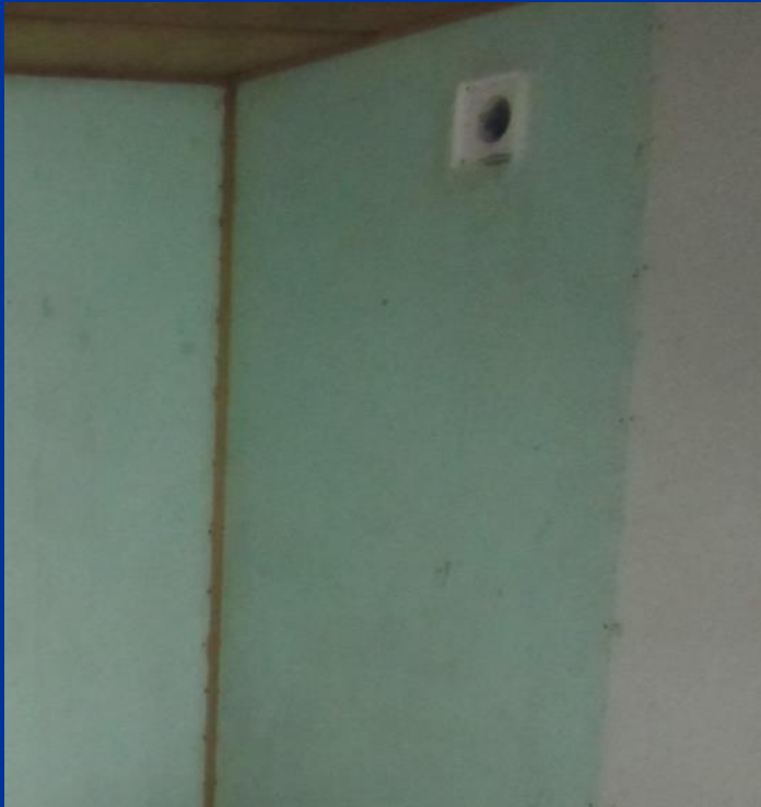
Ventilation intake plugged with a rag
