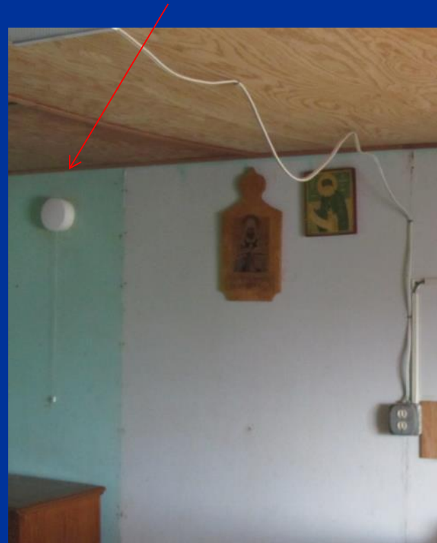
New ventilation intake
