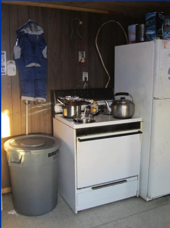
Cooking stove with no range exhaust
