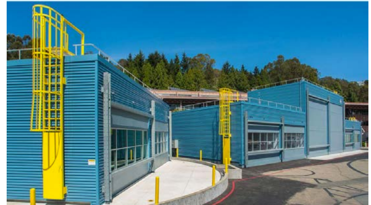
FLEXLAB Facility at LBNL
