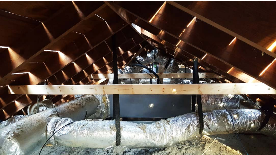
Collar-tie reinforcement
