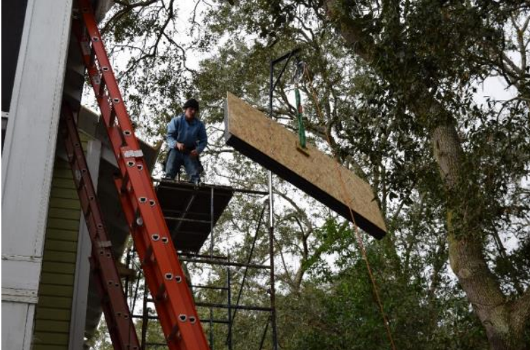
Lifting a nail-base panel
