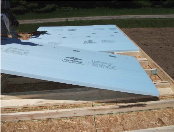
Foam is installed against an extended bottom plate
