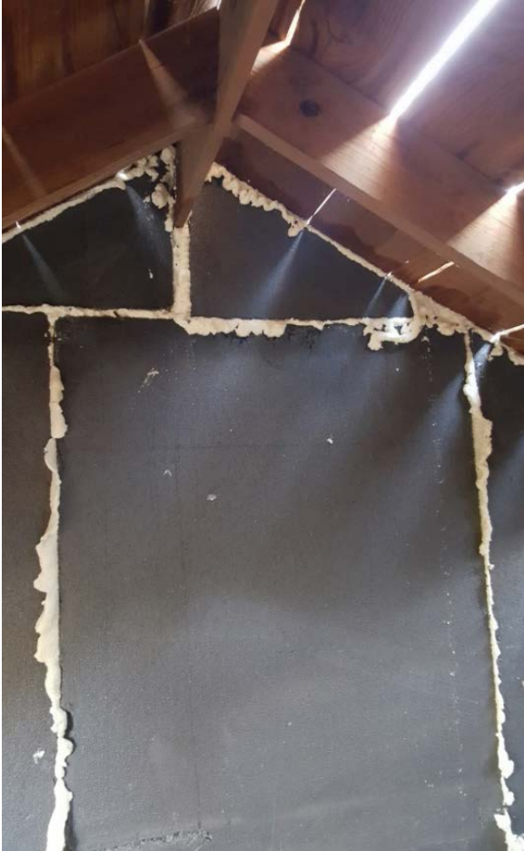
Gable Wall Insulation
