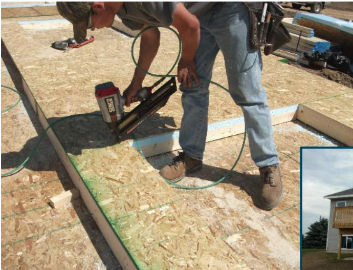
OSB is nailed over foam sheathing
