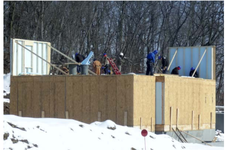
Standard OSB Exterior, Stud Cavity, Foam Interior
