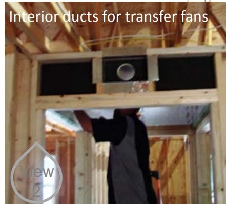
T-Fan 1 T-Fan 2 Interior Ducts
