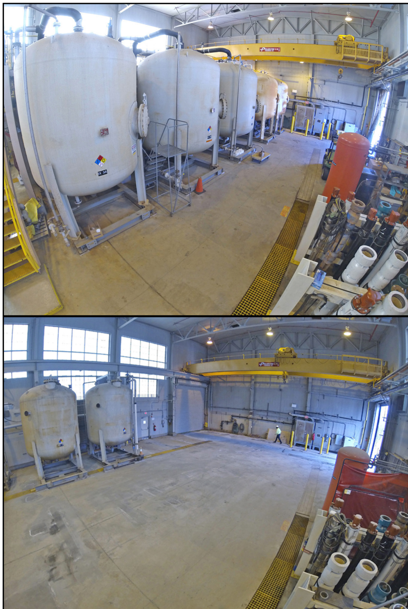
CAWWT interior before (October 2016) and after (January 2017) tank removal to provide room for the new, smaller treatment system.
