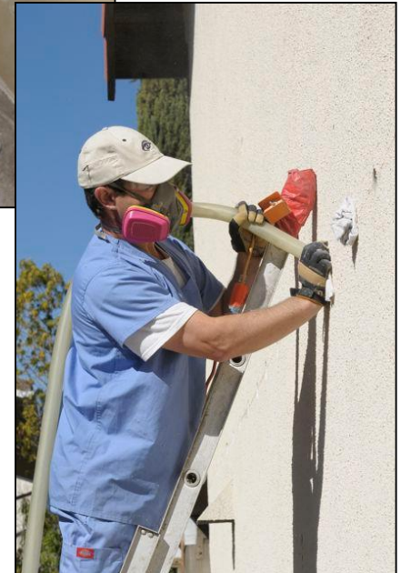
Option 2: Exterior drill-and-fill
