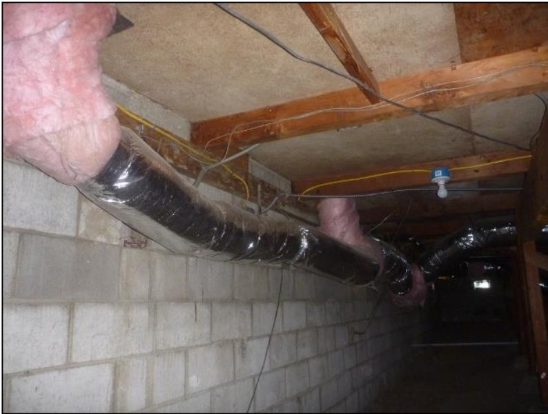
Before Example: Floor Joists without any insulation
