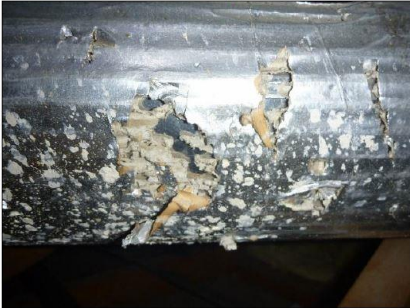
Friable asbestos wrapped ducts:
