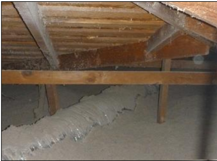
Partially exposed air duct
