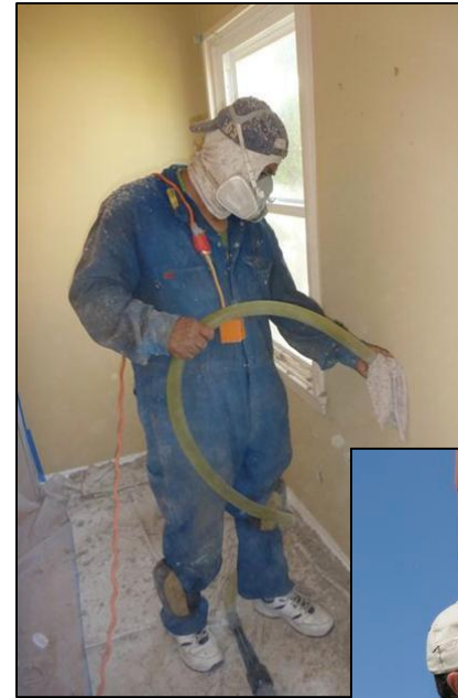
Option 1: Interior drill-and-fill
