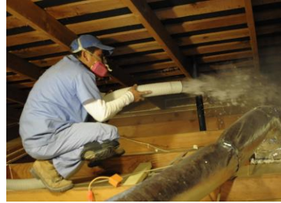
Blown Insulation
