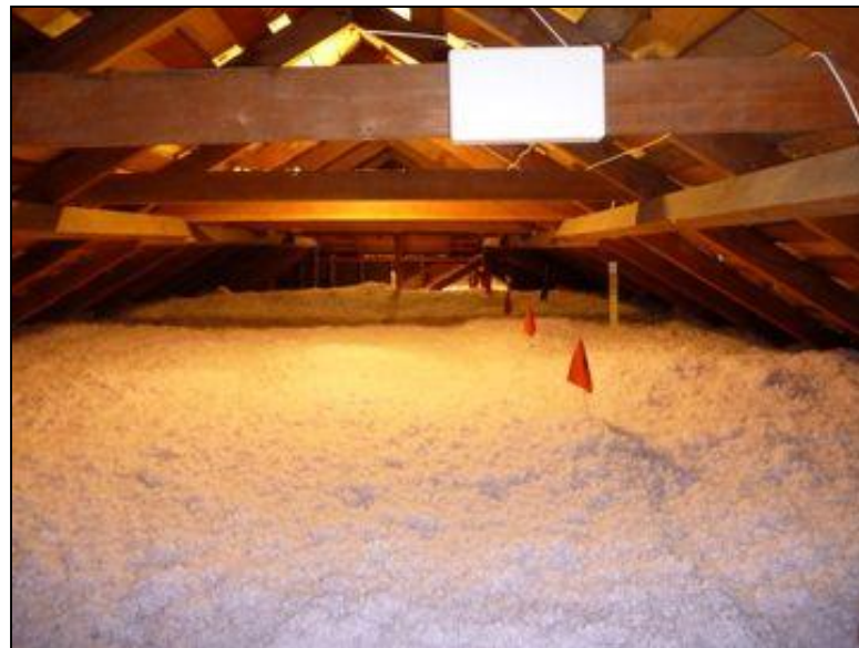
After Example: Attic with R-38 blown in insulation, ID flags and attic rulers
