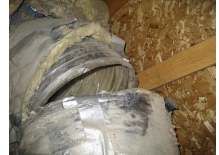
Duct Sealing or Replacement
