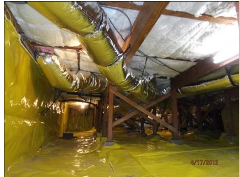
After Example: Crawl space with VOC-free batt insulation beneath the floors and a moisture vapor barrier
