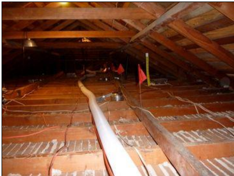
Before Example: Attic with no insulation
