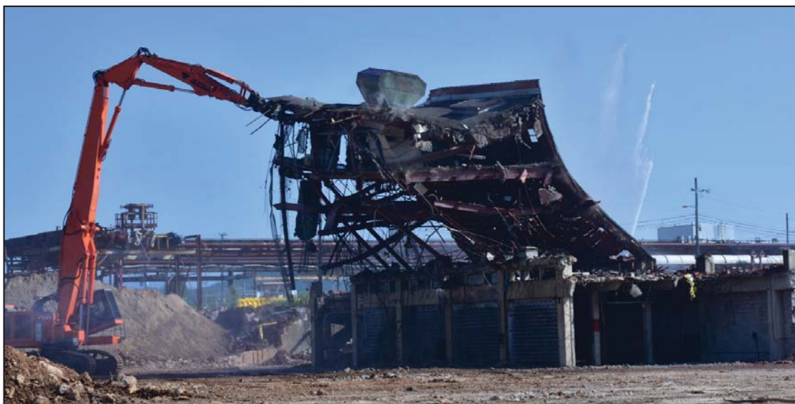
The demolition of K-27 at ETTP marked the historic end of an effort to remove all gaseous diffusion buildings from a single site.
