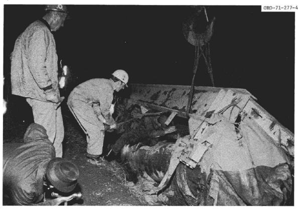
Fig. 4-4. Initial lift during cask retrieval (Chandler 1972).
