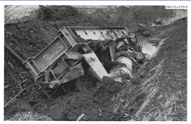
Fig. 4-1. Hallam cask embedded in ditch after accident (Chandler 1972).
