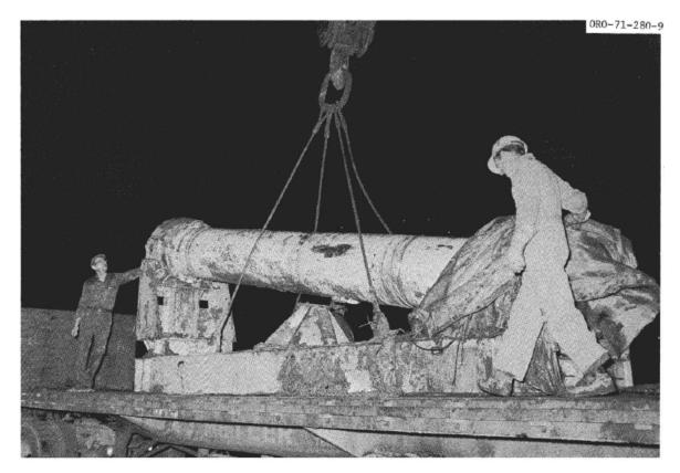
Fig. 4-5. Cask placed on trailer (Chandler 1972).
