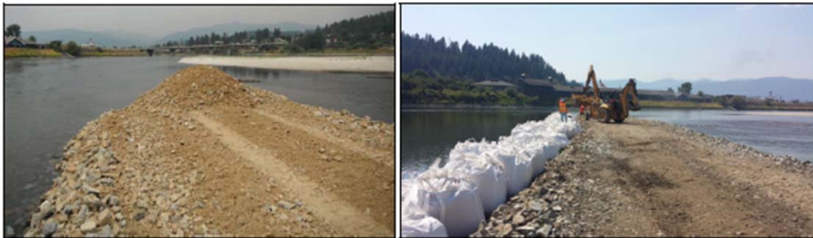
Figure 9 Examples of temporary river access road construction
