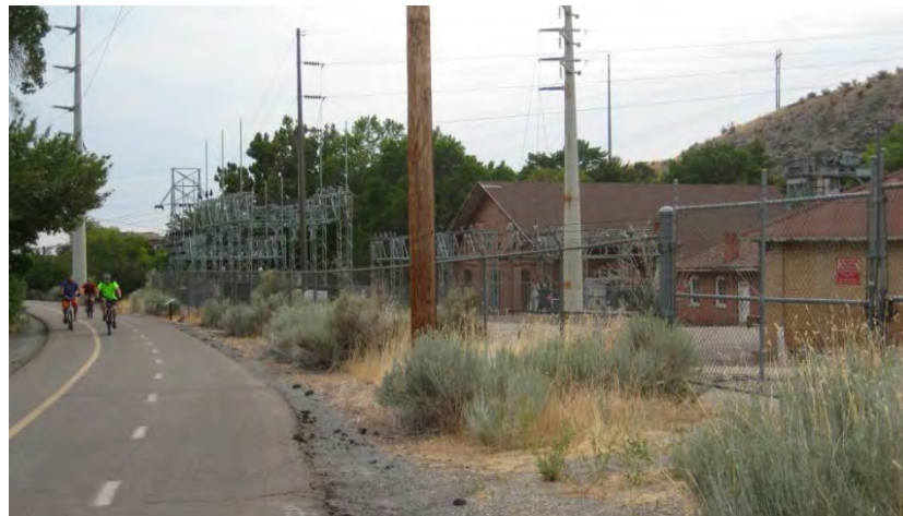
View of Olmsted Power House and Auxiliary Buildings from the Provo River Parkway Trail
