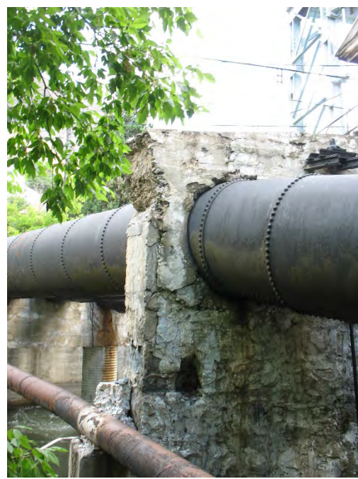
Concrete deterioration on penstock supports
