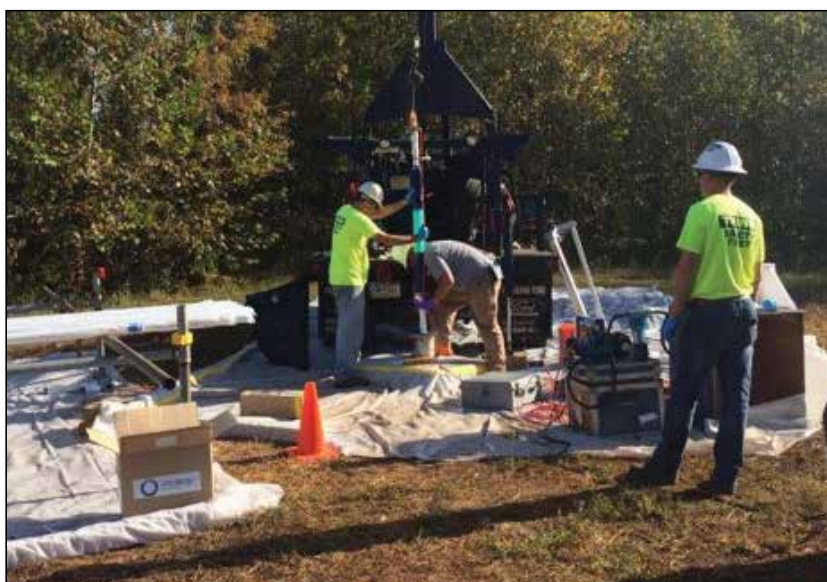
Workers install a Westbay™ discrete zone groundwater sampling system in a deep monitoring well in Melton Valley. This type of sampling equipment allows sampling at very specific depth intervals in wells such as in individual fracture zones that may transport contaminated groundwater.
