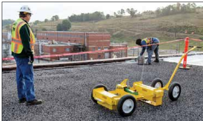
Workers repair the roof of the Alpha 4 Building at Y-12.
