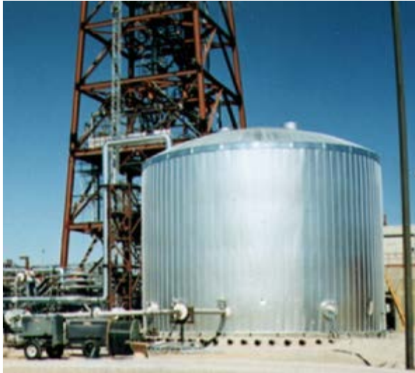
Externally insulated tank at Solar Two
