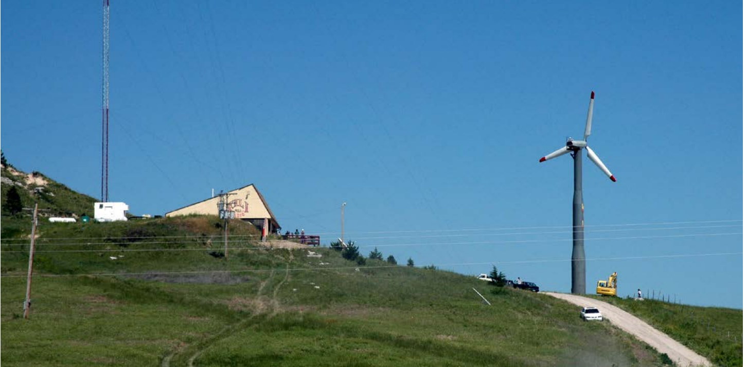
The U.S. Department of Energy's Office of Indian Energy provides financial assistance to federally recognized tribal governments and Alaska Native corporations to develop and deploy renewable energy projects on tribal lands. Shown here: a 65-kilowatt turbine supplies power to the Pine Ridge Reservation radio station in South Dakota. Photo by Bob Gough, NREL 16258
