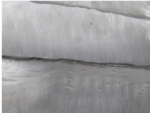
Figure 5: Grinding and machining marks associated with a circumferential weld. This treatment will significantly impact the near surface stresses associated with the processed regions.
