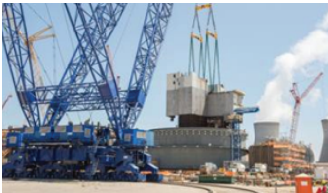
Vogtle Progress – Left: Placement of Unit 3 CA01 module; Right: arrival of Unit 4 make up tank (Courtesy of Georgia Power/Southern Company)
