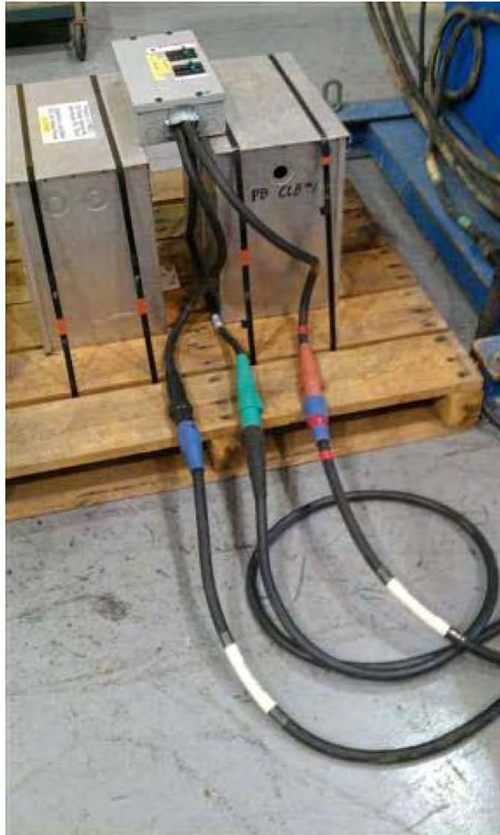
Capacitive load bank connections
