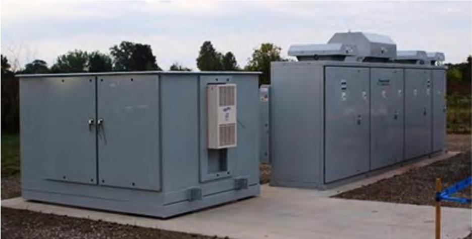
**Figure 9: 500 kW Battery on the right and PCS at MCCC**
