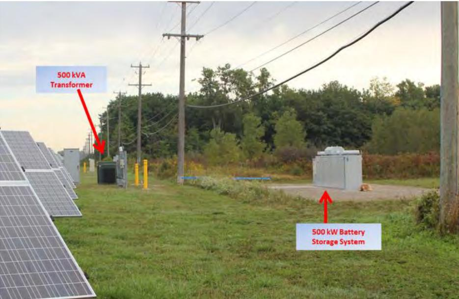
**Figure 10: Ground View of 500 kW PV and Energy Storage at MCCC**
