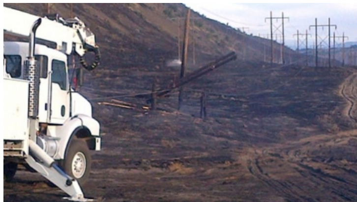
Figure B.2 Wildfire Damage to Electric Distribution System Wood Poles
