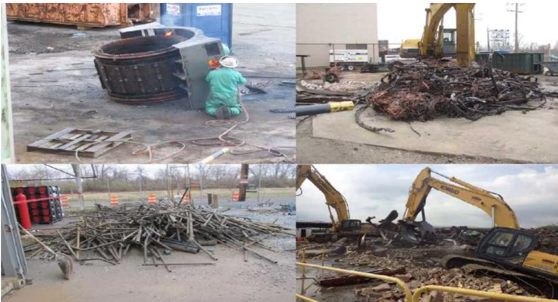
Photo 6.2. View of Salvage Operations to Harvest Non-Ferrous and Ferrous Material Following Power Plant Demolition 317
