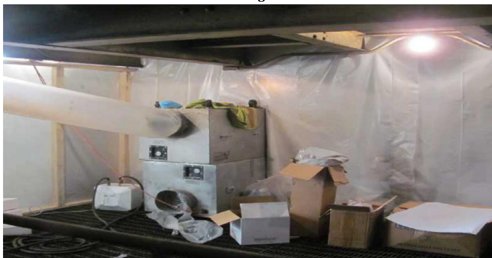
Photo 6.3. View of Asbestos Containment Area During Demolition 322
