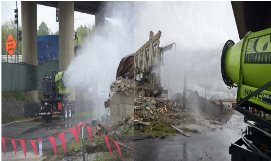
Photo 6.4. Management of Dust During Demolition 325
