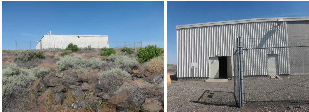
Figure 3-4. Views of the Pump House from the River (L) and from Parking Lot (R)
