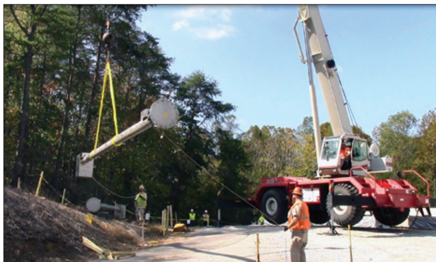
An MSRE salt probe is being positioned for nondestructive assay.
