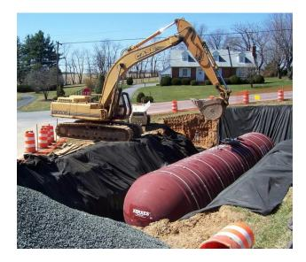
30,000 gallon underground tank contains 200 MWh (plus 600 MMBTU CHP heat
