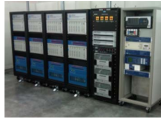
Electrolyzer integration with grid (INL/NREL)
