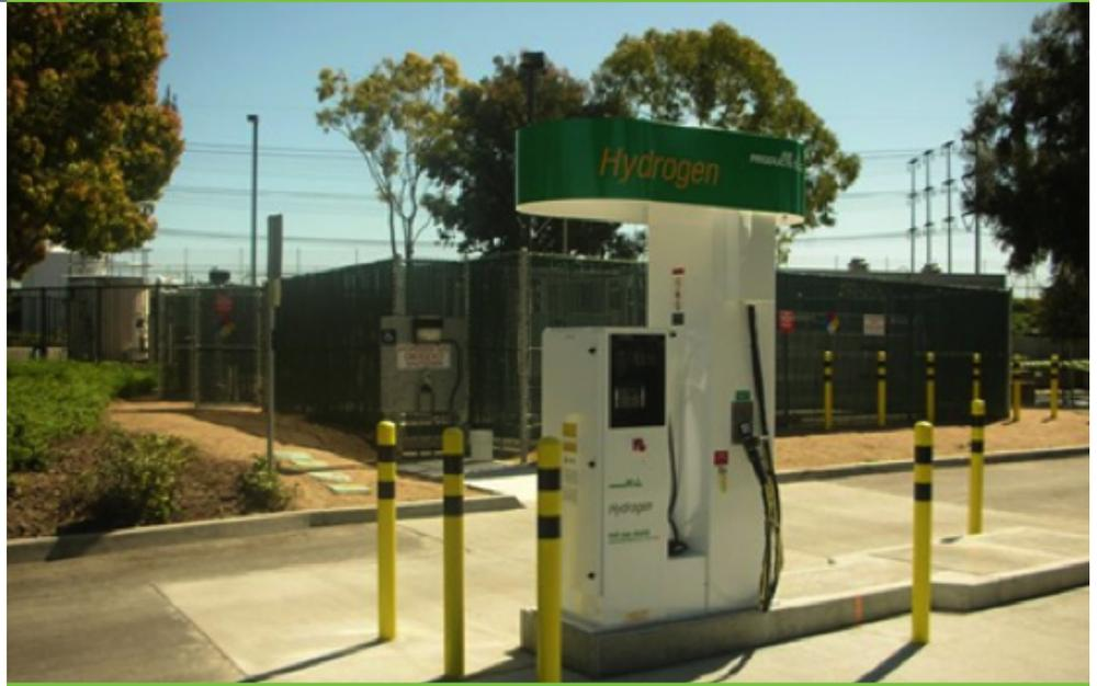
Photograph of the state-of-the-art hydrogen fueling station with fueling at 5,000 and 10,000 psi according to the latest SAE protocols for rapid 3-minute complete tank refueling.
