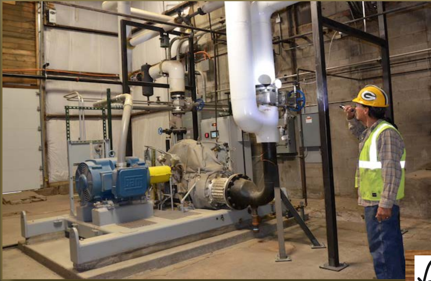
Backpressure Steam Turbine Generator
