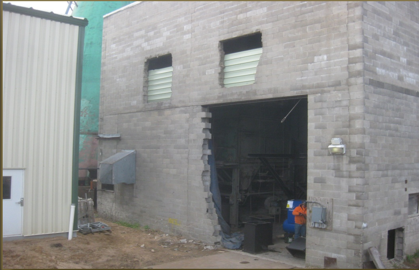
Demo old boiler
