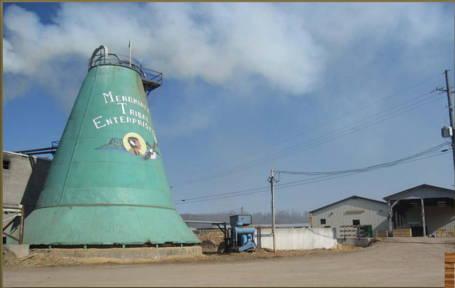
Old Fuel Processing and Storage
