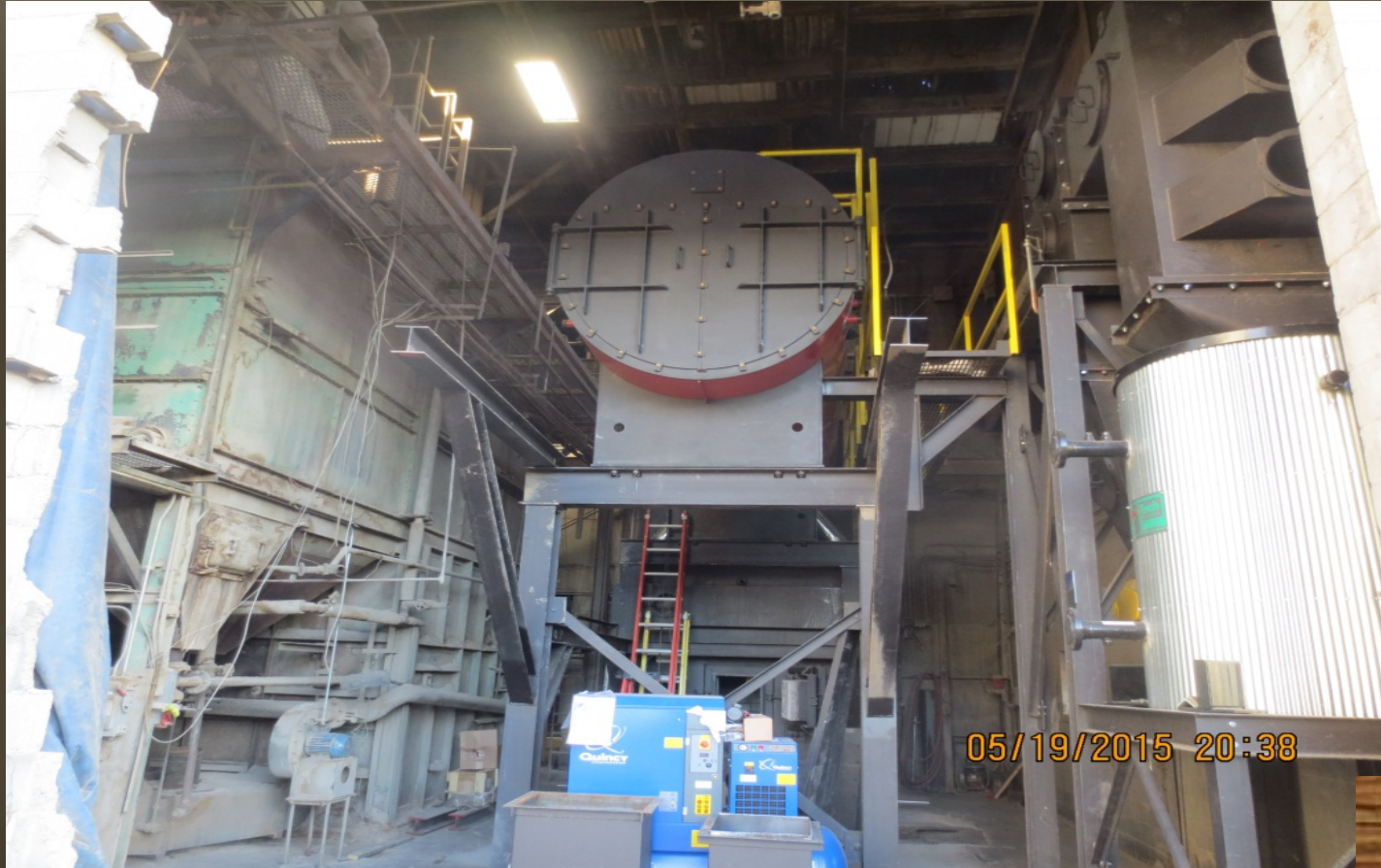
Installed new boiler
