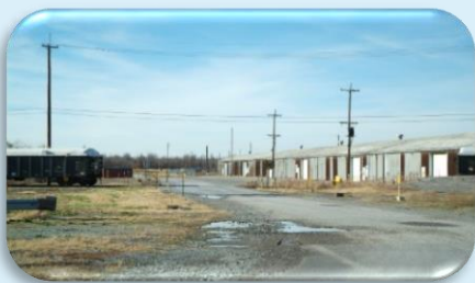
C-746-B warehouse before.
