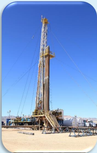
Groundwater characterization well ER-3-3 was drilled to a depth of 3,193 feet below the ground surface of Yucca Flat in February.
