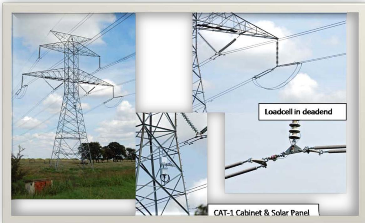
**Figure 15 - 345 kV CAT-1 Installation**
