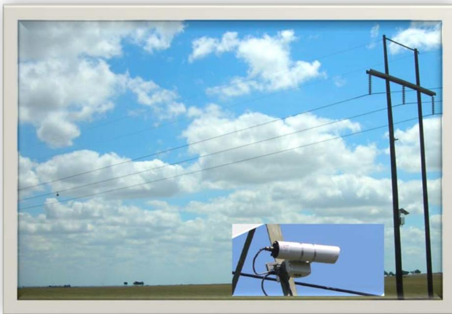
**Figure 17 - Sagometer Installation on 138 kV Wood H-frame**
