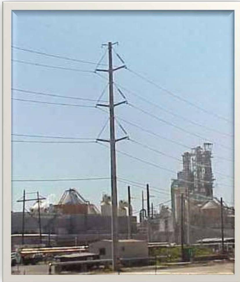
**Figure 14 - Suspension Structure**
