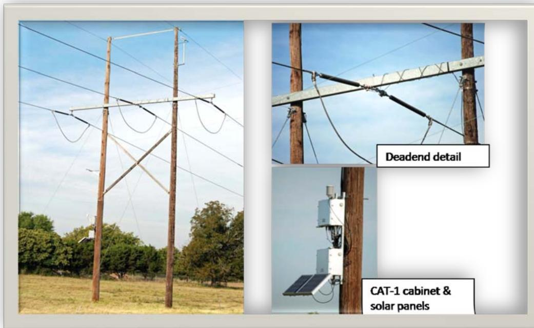
**Figure 16 - 138 kV CAT-1 Installation**
