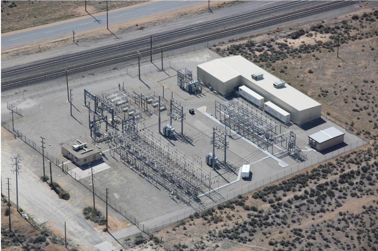
**Figure 3-1** Monolith Substation and BESS Facility
