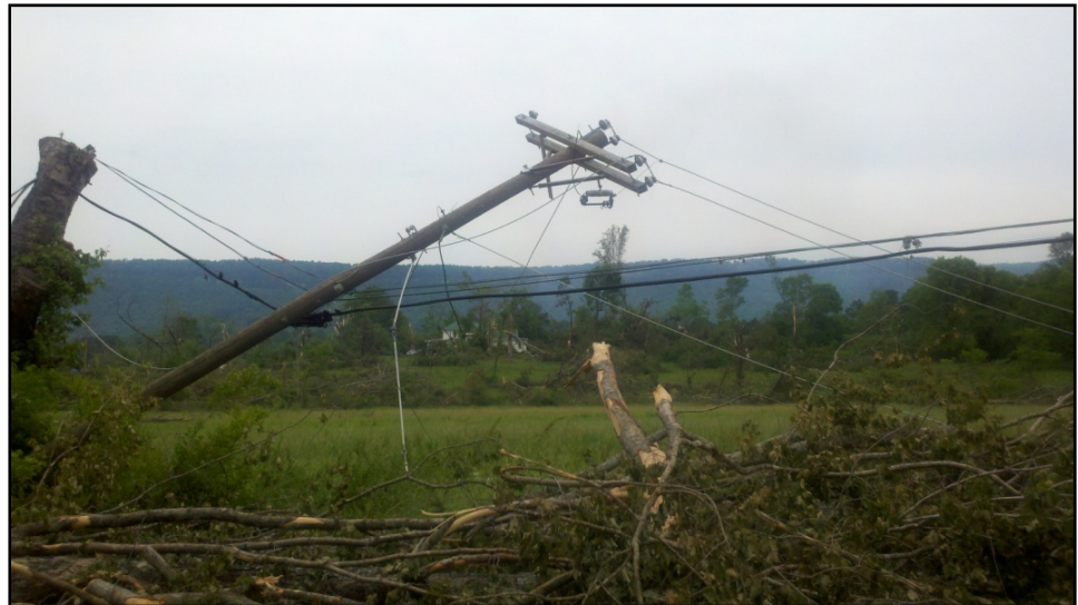
Downed power line as a result of April 2011 storm
