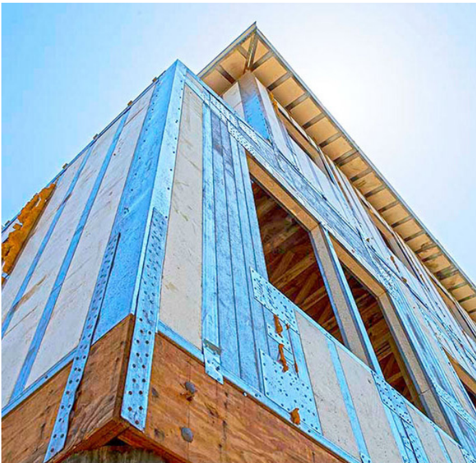
High-performance wall panel construction in Johns Landing, SC. Image courtesy of Insulsteel Building Enclosure.
