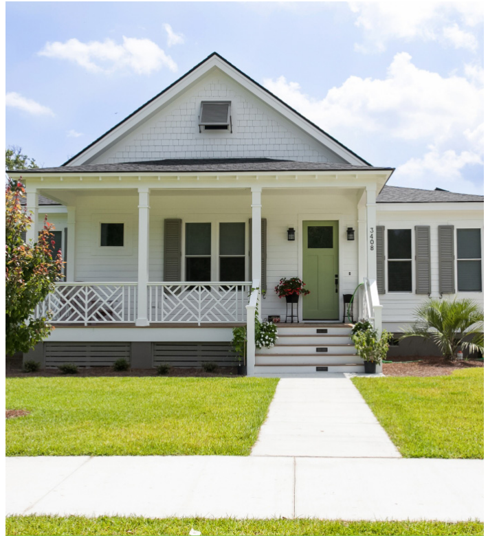
Zero Energy Ready Home in Charleston, SC. Image courtesy of Amerisips Homes, LLC.
