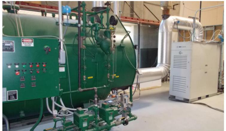
The FlexCHP-65 system consists of Johnston Boiler Company 100-horsepower firetube boiler, GTI-developed supplemental Ultra-Low-NO<sub>x</sub> burner, and Capstone C65 microturbine.
