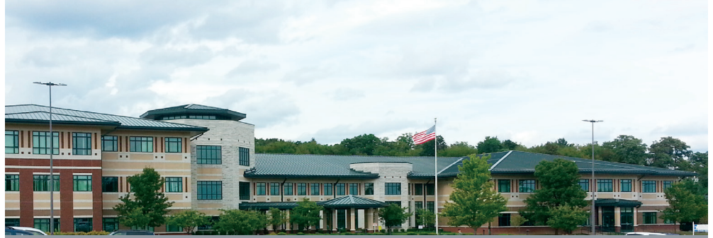
The Technical Sergeant McGarity Army Reserve Center located in Coraopolis, PA, replaced over 1,250 troffers in three buildings and achieved an impressive 51% energy savings, or 184,000 kWh annually. The Army Reserve is proud to contribute to the efforts of the Interior Lighting Campaign, which have saved over 130 million kWh and $13.5 million in the first year.
