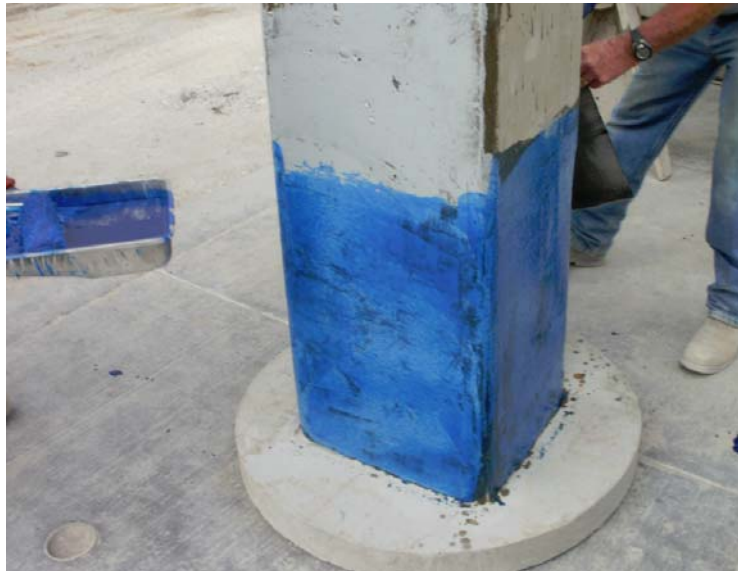
Figure 11B – Saturant Application
