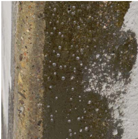
Figure 5B – Outgassing Following Primer Application
