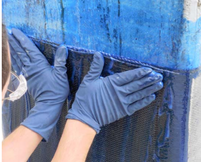
Figure 16B – Positioning the Carbon Fiber
