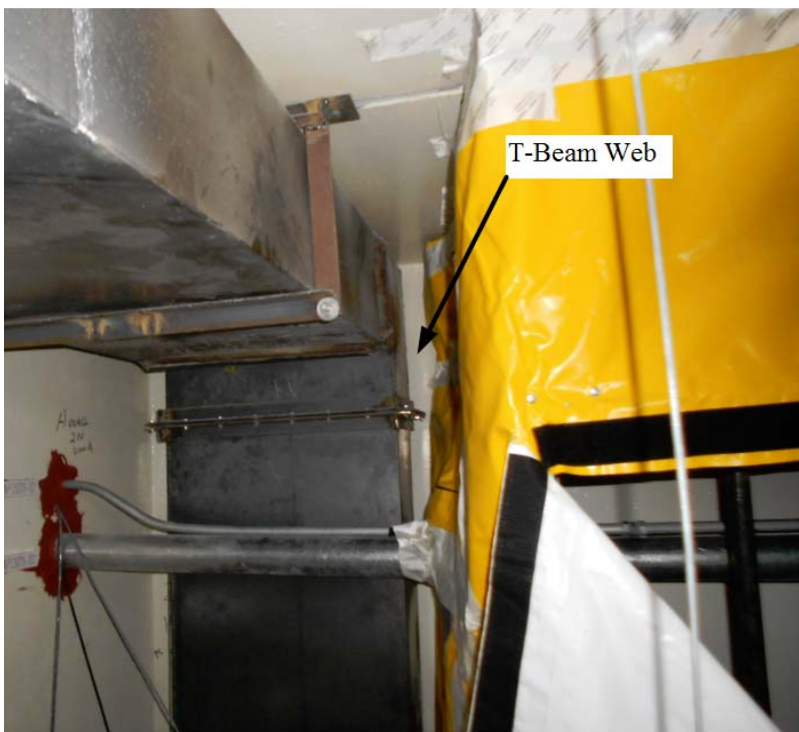
Figure A5A – Obstructions at Girder to Receive FRP
