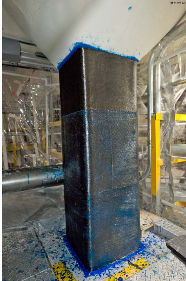
Figure A3 – Circumferential Jacketing of Columns in PF-4
