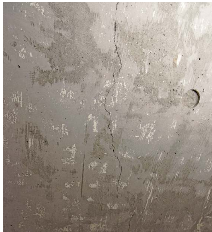
Figure A22 – Typical Crack in Concrete Substrate
