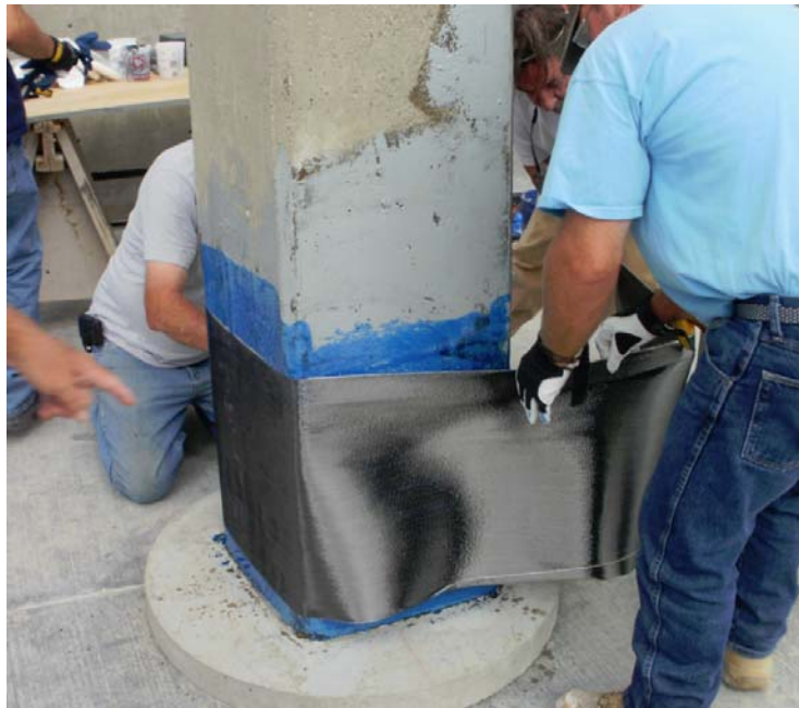
Figure 13B – Carbon Fiber Installation
