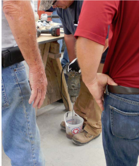
Figure 2B – Mixing of the Primer
