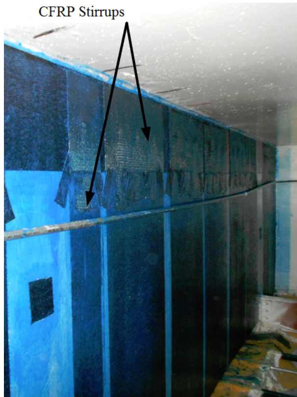
Figure A4 – CFRP Reinforcing on Web of PF-4 Roof T-Beam
