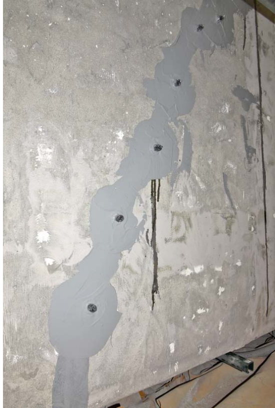
Figure A23 – Epoxy Crack Injection
