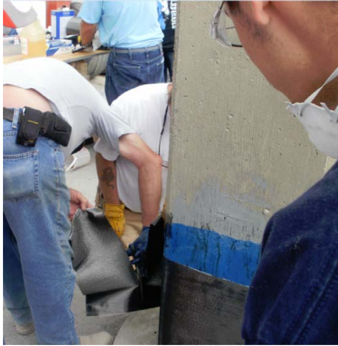
Figure 14B – Cutting of Carbon Fiber with Scissors
