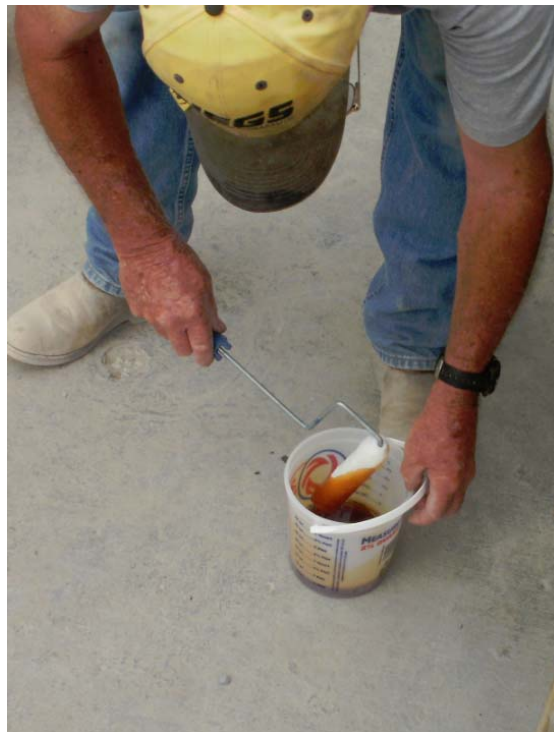
Figure 3B – Preparing to Apply Primer
