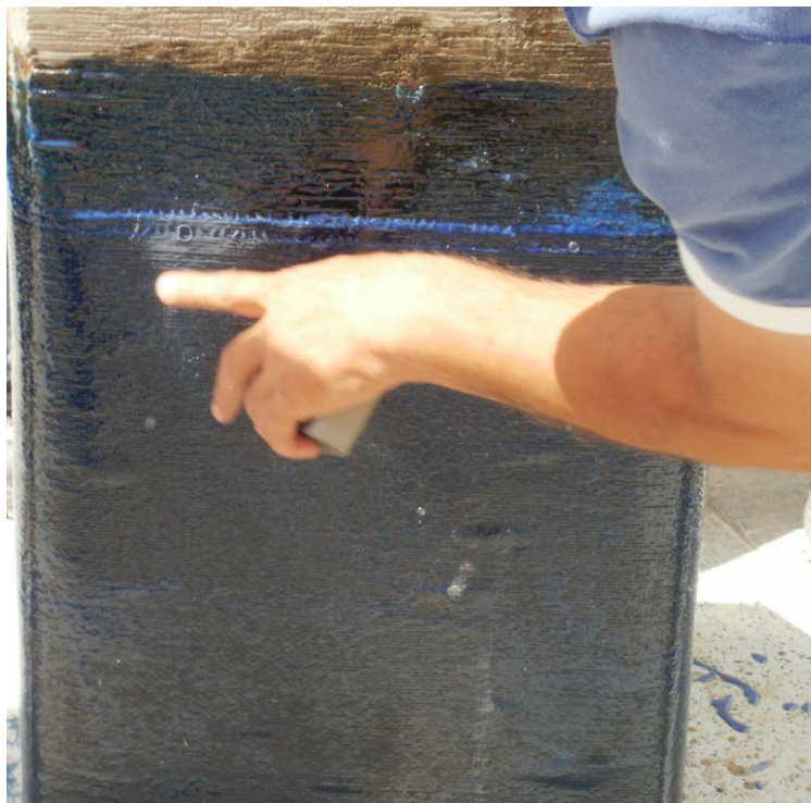
Figure 19B – Sanding of Outgassing Bubbles on Cured FRP
