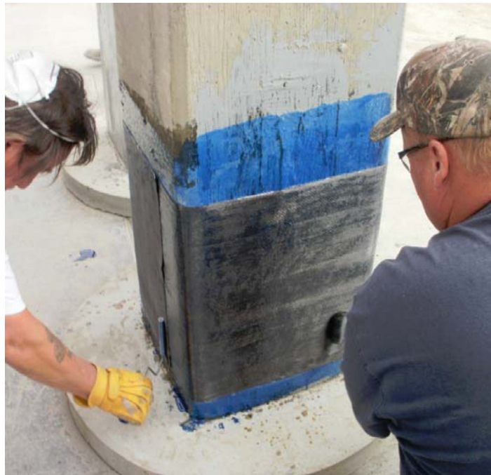
Figure 17B – Rolling Carbon Fiber into Saturant
