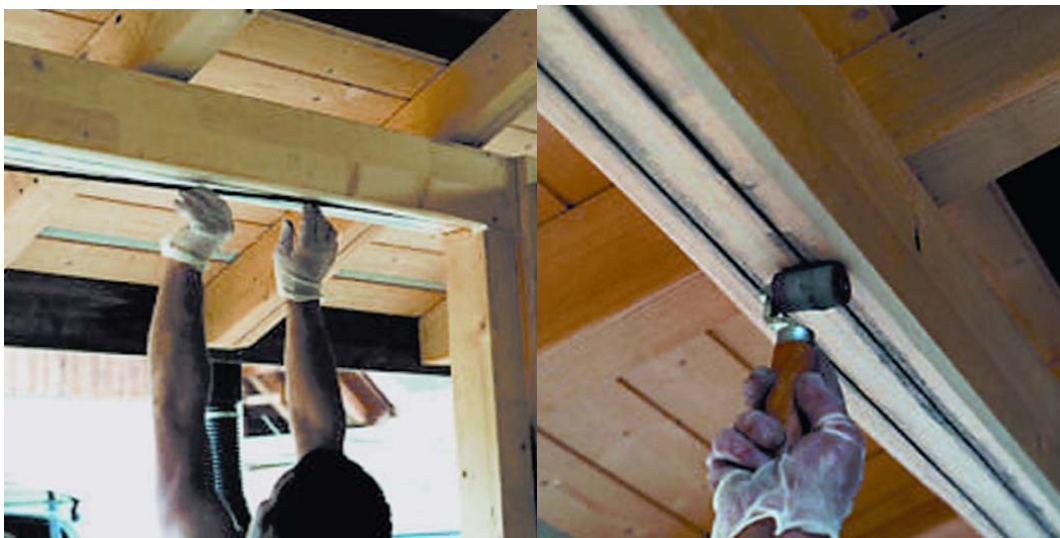
Figure A10 – NSM in Timber Beam 1
