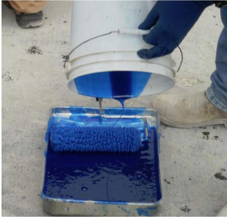
Figure 10B – Preparing to Apply the Saturant
