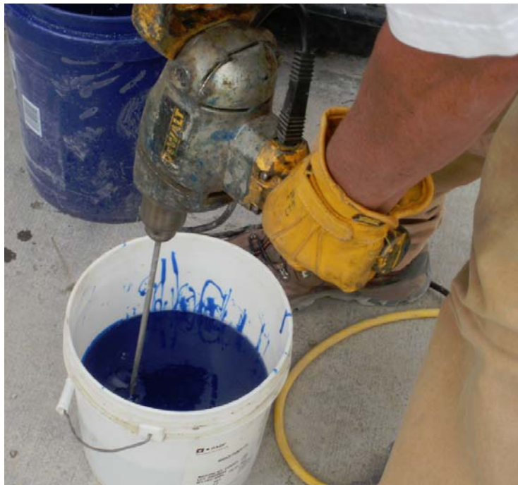
Figure 9B – Mixing of the Two-Part Saturant
