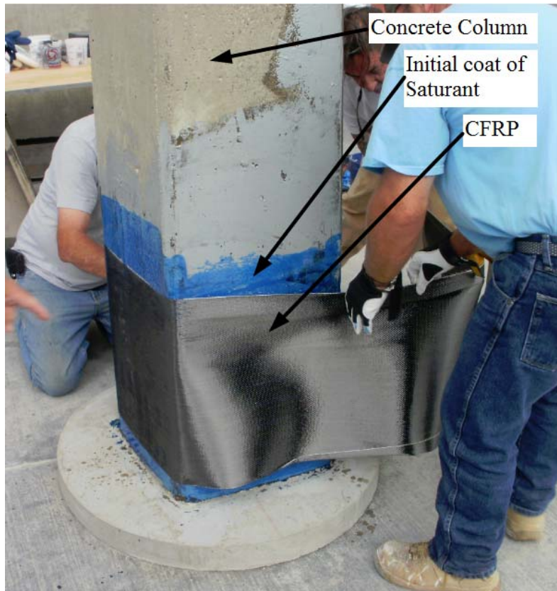
Figure A1 – Wet Layup Process
