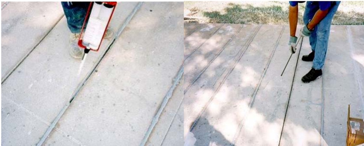
Figure A2 – Near Surface Mounted (NSM) FRP 1
